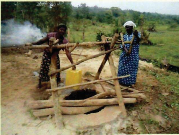
Fig 16: A Shadoof well from which farmers collect water for their nursery bed
