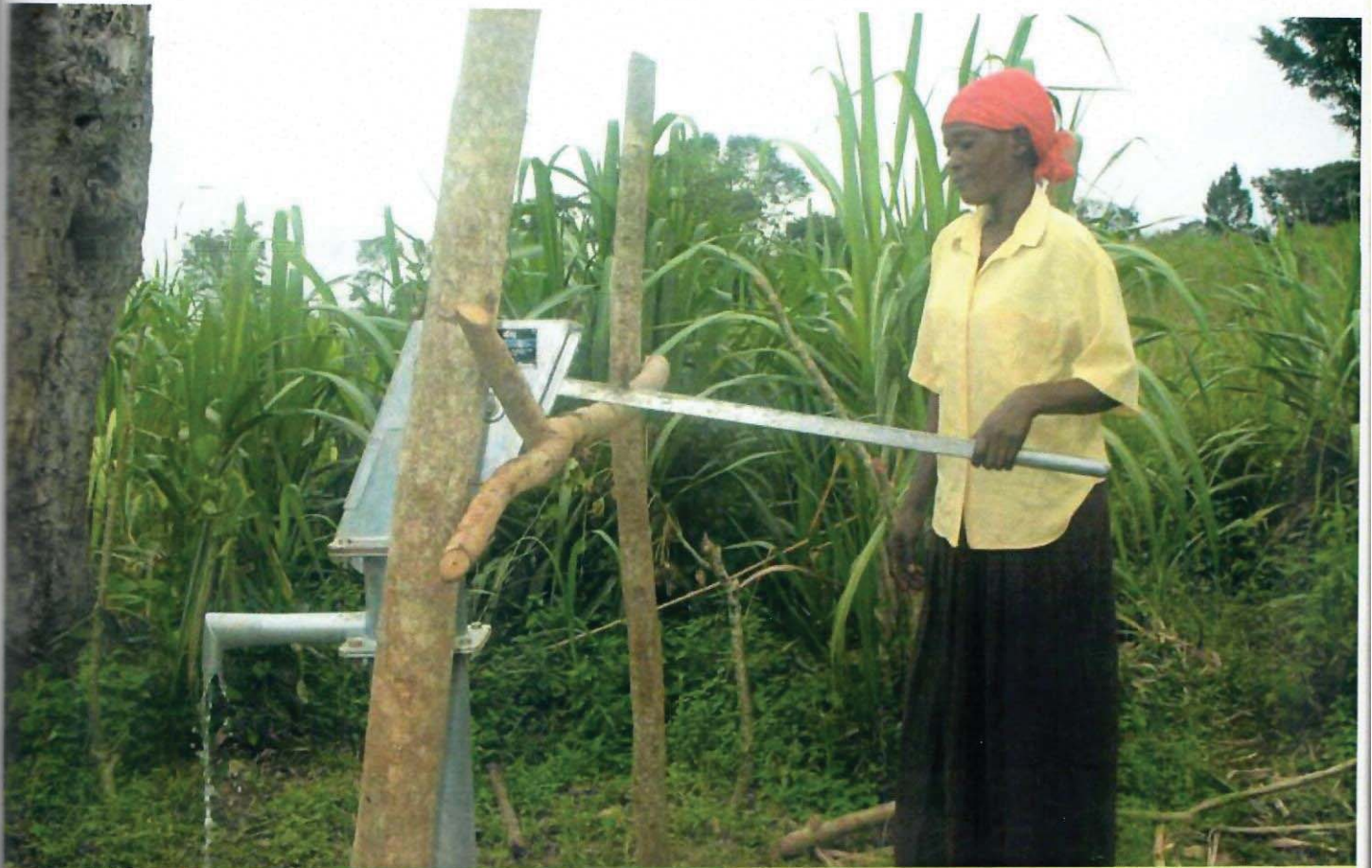
The new well constructed with support from the project. 'The new well will protect us from water borne diseases, thanks to the project' says Ms. Nampijja.
